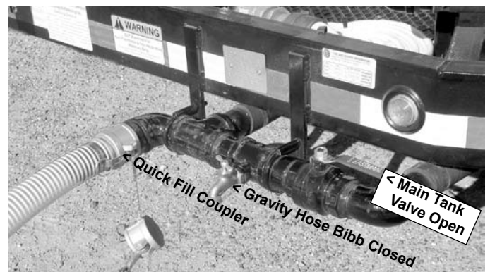
Figure B4 Filling Tank With Transfer Pump
