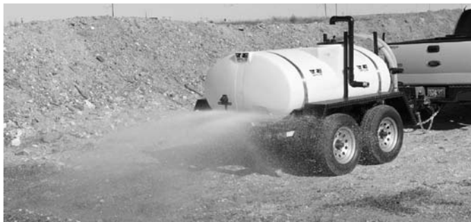
Figure B9 Operating Spray Bar
