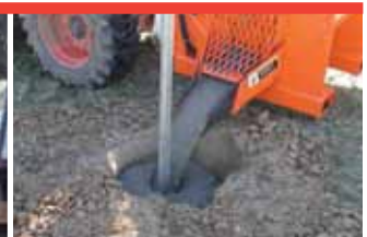
After mixing, unload right where it is needed. No unnecessary steps.
