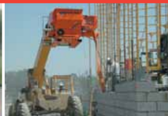
Grout using only two people
